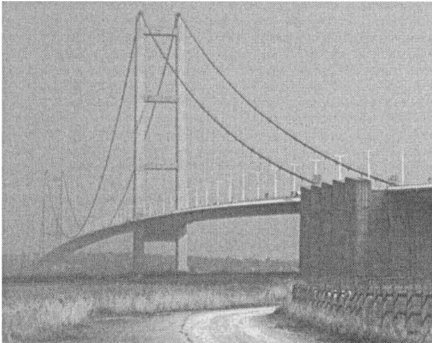
Figure 2.3 Humber Bridge (Reproduced by kind permission of The Humber Bridge Board)
